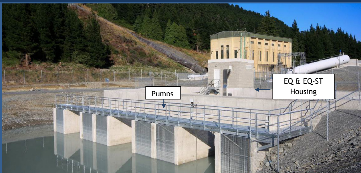
Figure 1: BCI Pump House Irrigation Site
